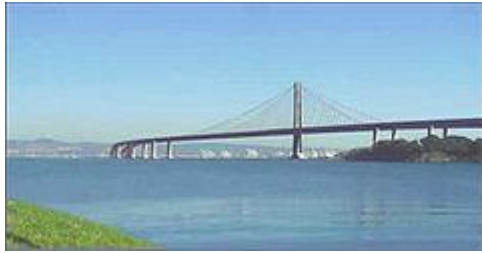
Eastern span replacement of the San Francisco – Oakland Bay Bridge
